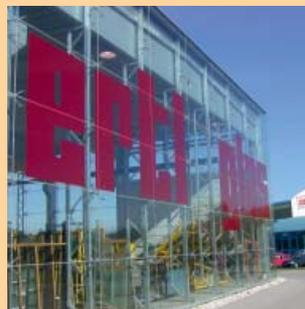
Facade from ertex ESG attached by points to a steel construction.
