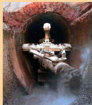
MCS Inliner - Angerlehner sewer milling machine "AKF 40" at work.
